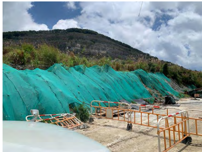
Impermeable cover for slope at System A.
